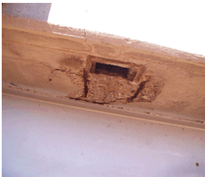
Figure 5-2. Corrosion damage due to concentrated de-icing solution at drain site.
