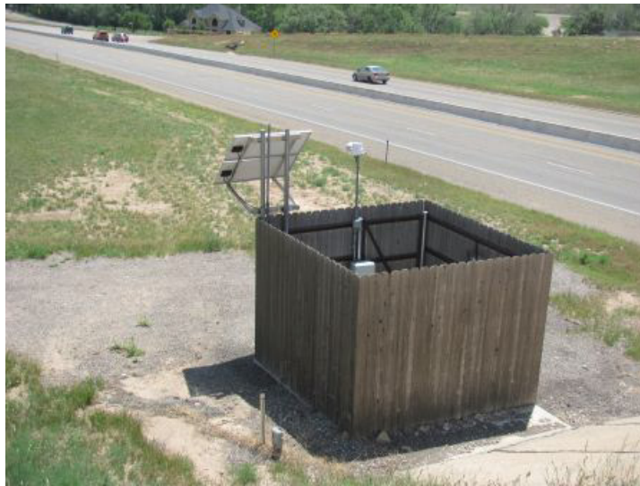
Figure 9-4. One means of achieving anti-icing is this automatic injection system in use in the Amarillo District. Photo shows chemical tank and controls, while the plumbing that gets the liquid to the road is underground.
