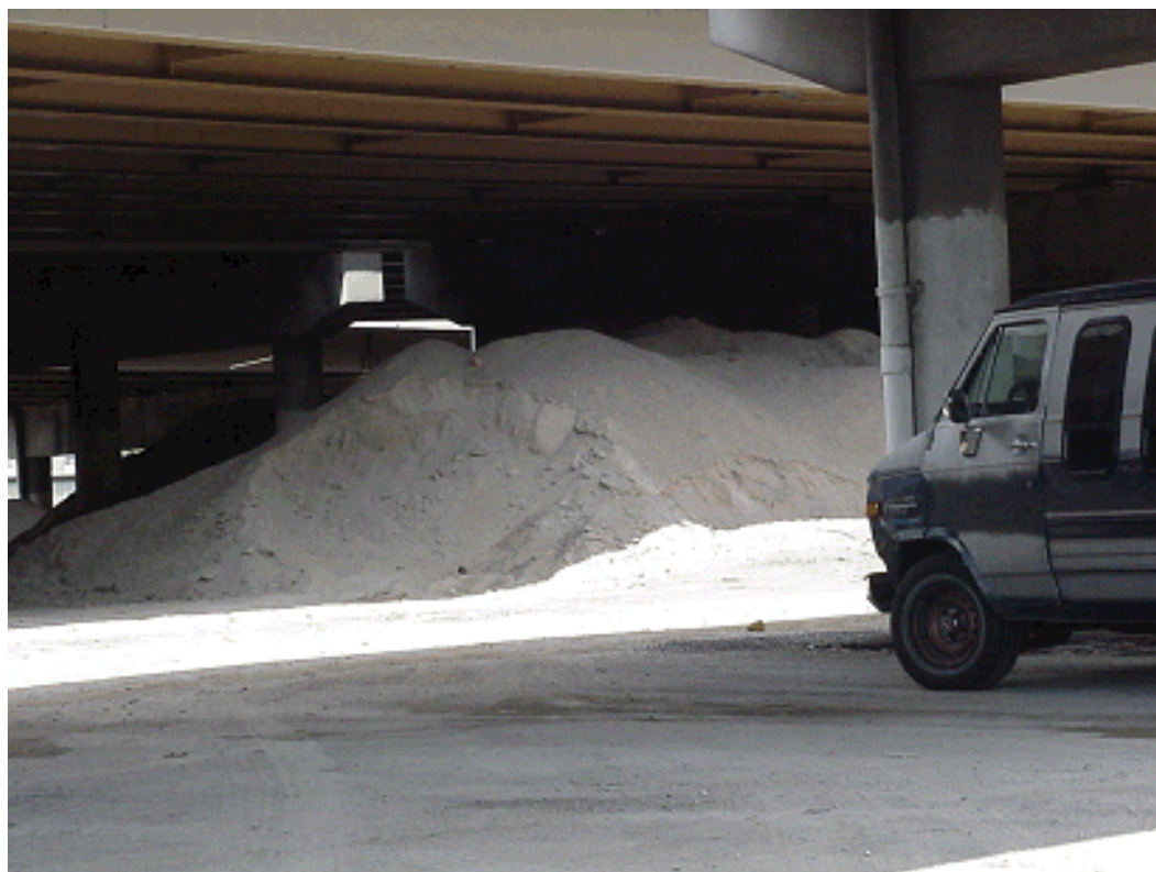
Figure 5-11. Salt storage under a bridge next to bridge columns.
