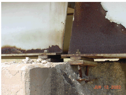
Figure 5-8. Failure on cap due to corrosion damage. Bridge was closed until repair could be performed.
