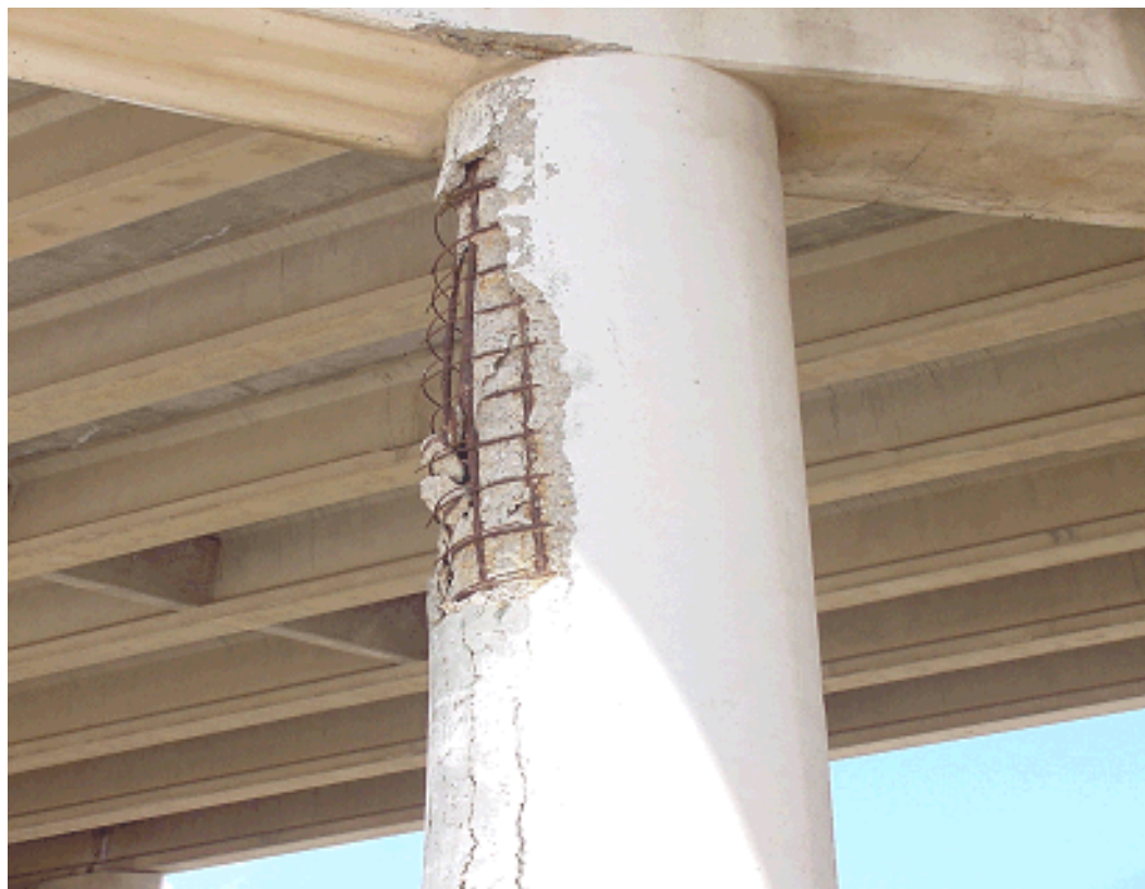
Figure 5-9. Column deterioration from chemical solution contamination.
