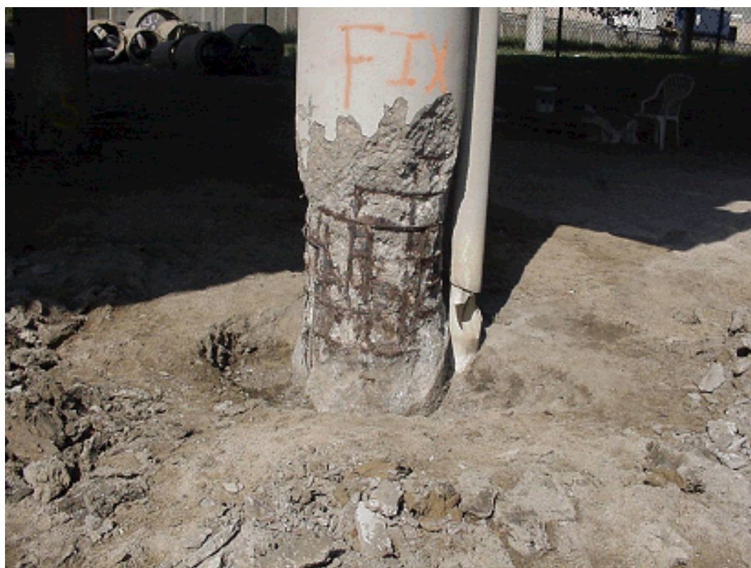
Figure 5-12. Damage created due to the salt storage.
