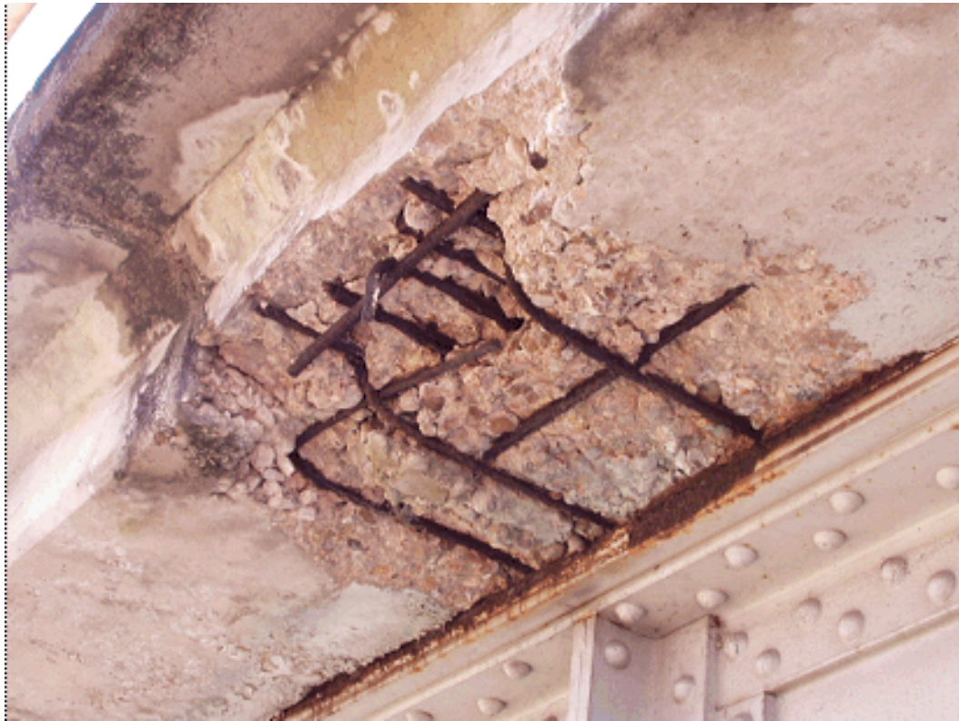
Figure 5-4. Poorly maintained joint allowed de-icer solution to damage overhang to second mat of steel and top plate steel on beam.
